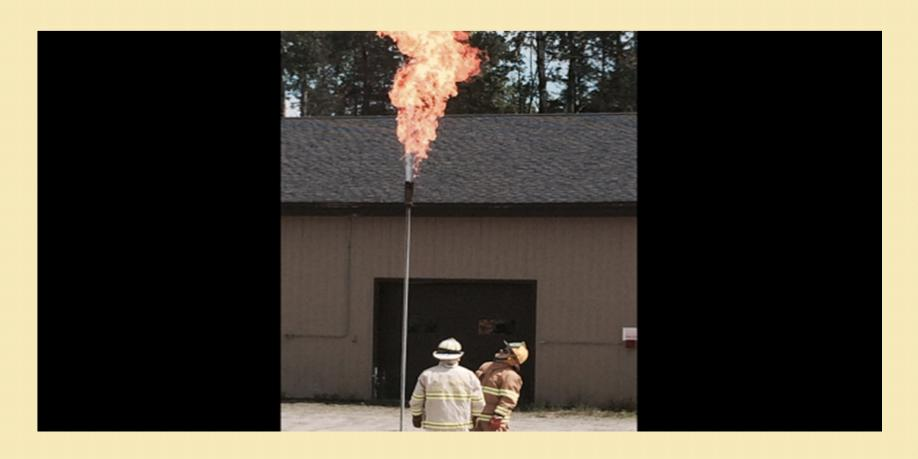
The flaring off of propane to reduce the pressure in a propane tank which needs to be evacuated of product. In some cases the gas is burned off to reduce the pressure in the tank so a leak can be stopped or safely repaired.
