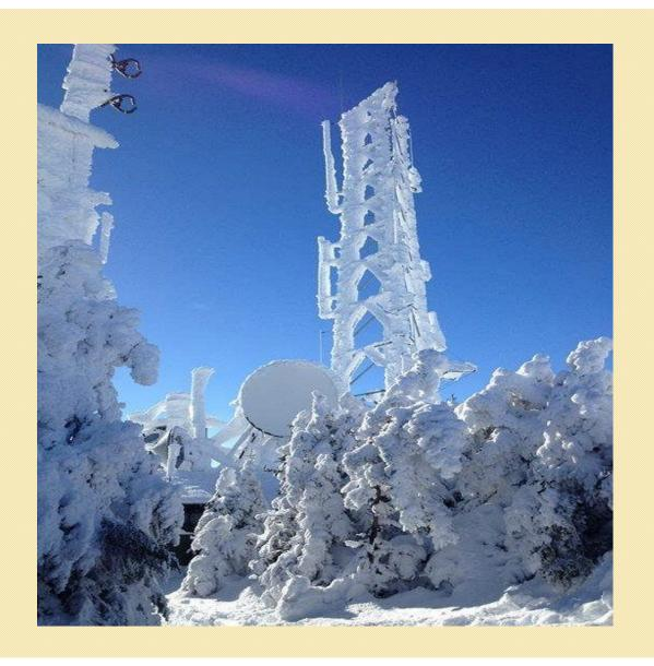
The summit of Killington receives frequent and heavy winter storms that coats our towers in a thick heavy blanket of snow and ice. These storms often contain dangerous wind speeds and brutally cold temperatures; factors that make servicing the equipment virtually impossible.
